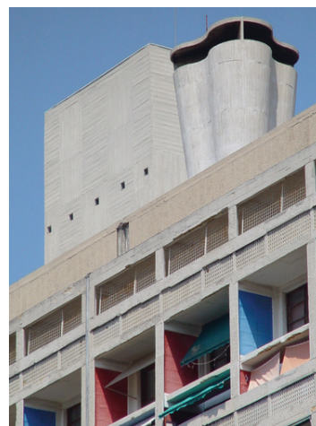
Figure 15 – Chimney for ventilation and view over the last floor verandas
