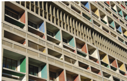
Figure 9 – Detail of the façade with vertical louvers at the 3d floor
